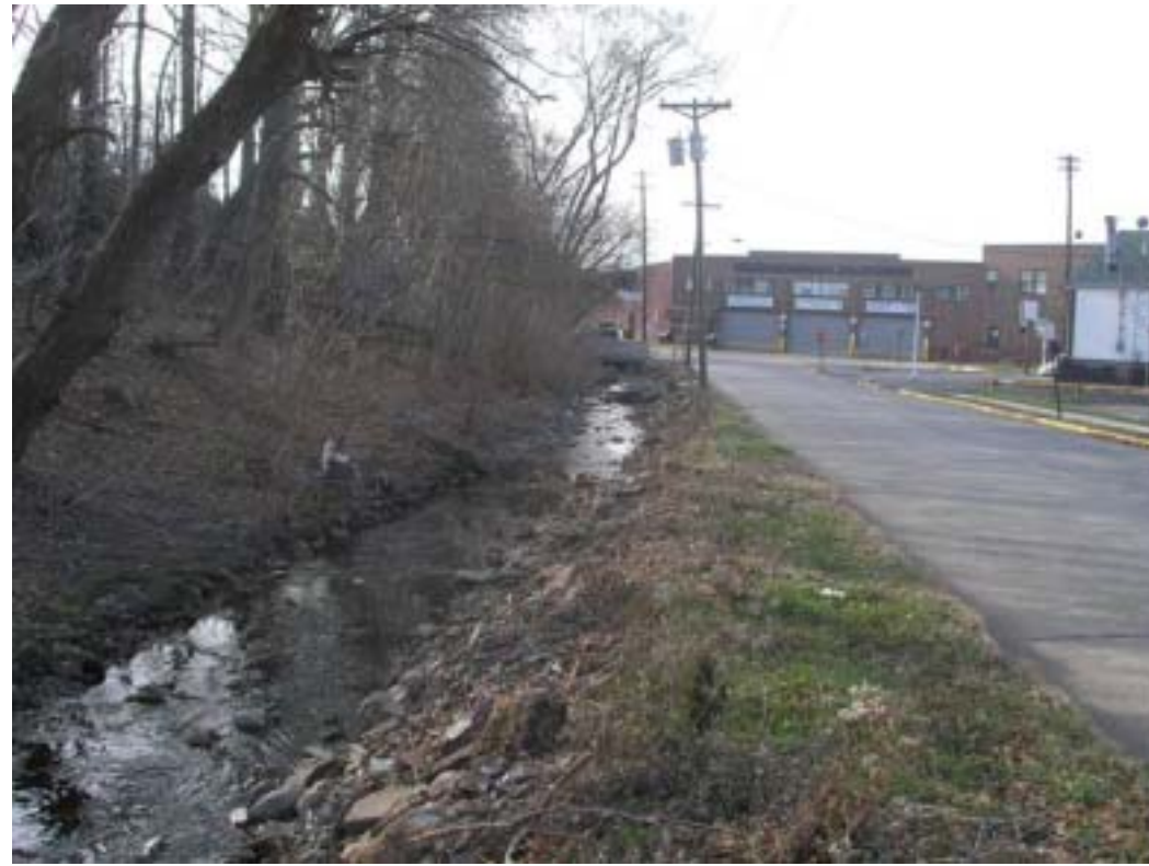
Elm Ave. creek dredged and cleaned.
